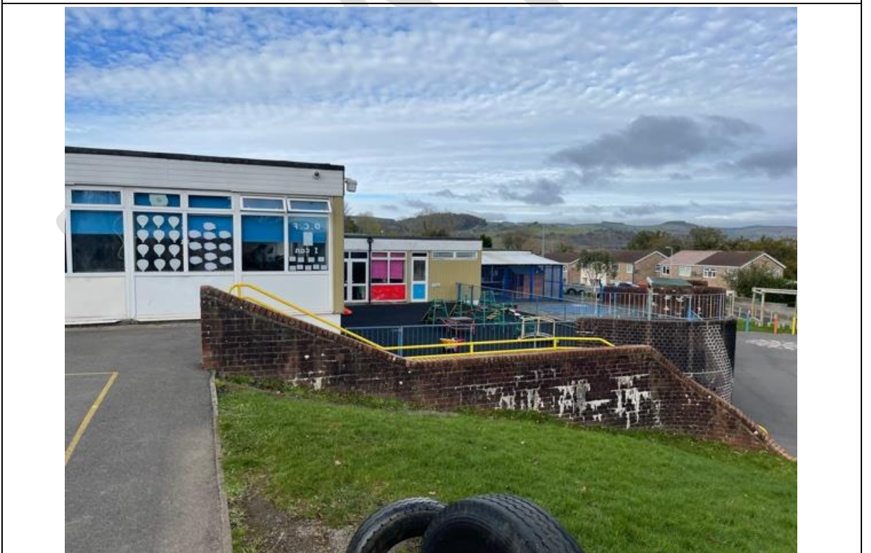
View of the school building from the Junior yard.
